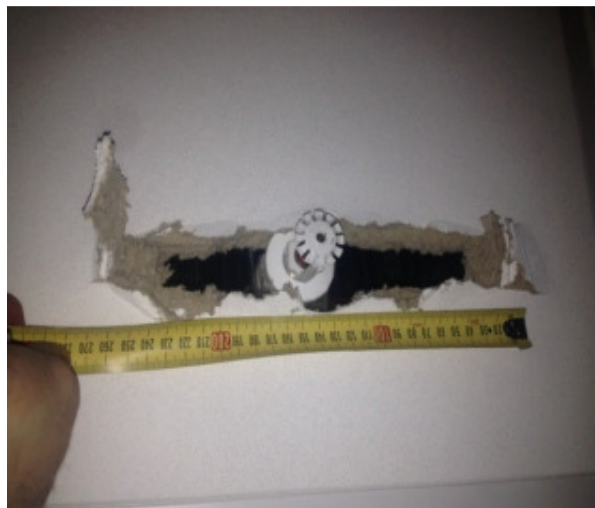
Figure 10: Relative movement of sprinkler and ceiling
