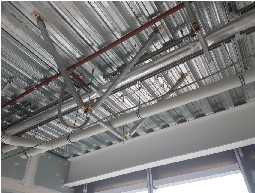
Figure 3: Seismic Restraint of services
